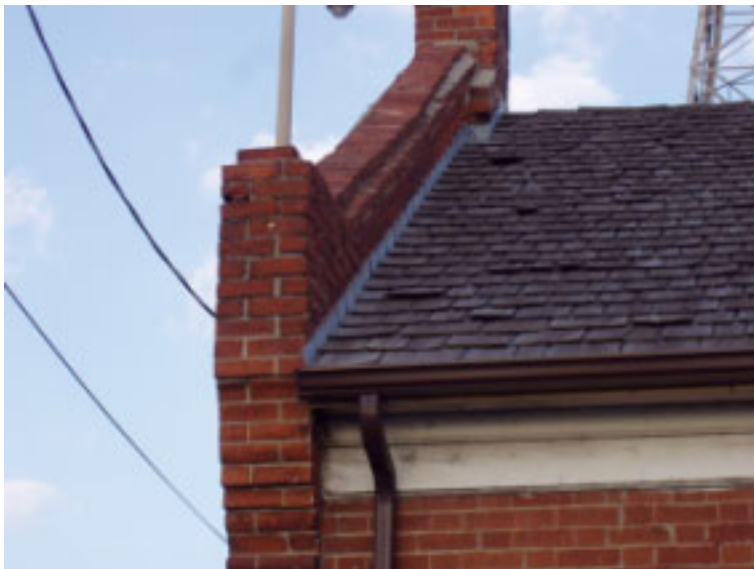
Detail of north gable. Note the shoulder under the chimney which is the base of the original chimney.
