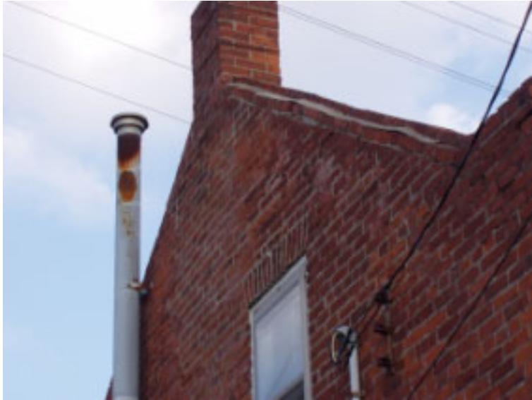
Gable wall – note the absence of a cap on the parapet and the small masonry chimney
